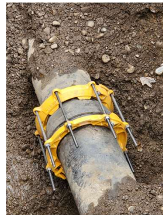
Repair Coupler on Cast Iron
